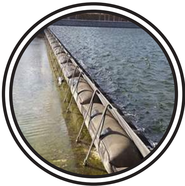
3. INFLATABLE BARRIER
