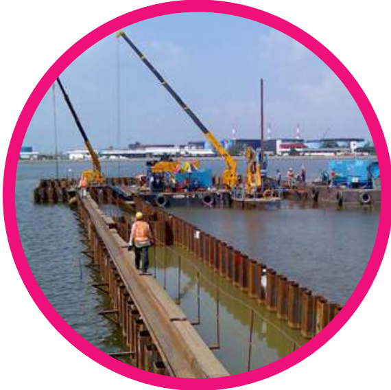
1. CRIBBING + SEALED SHEETPILES
