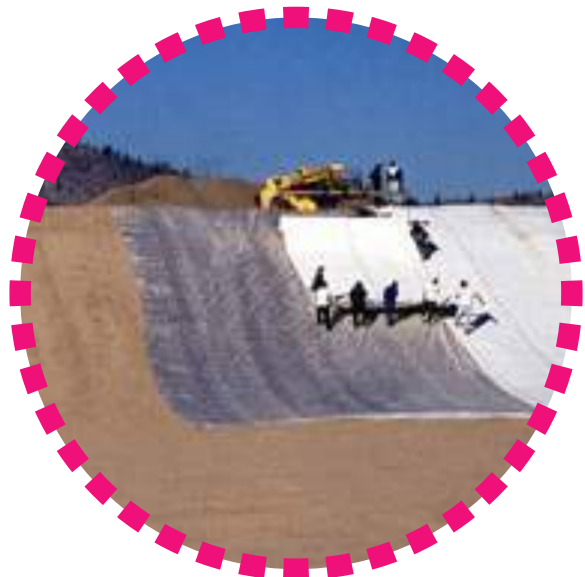
4. BENTONITE CLAY LINER
